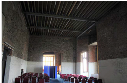
Modern ceiling structure visible throughout the ground floor - modern steel joists and timber rafters with plywood panels above
