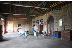
Part infilled door between the west range and main stair hall
